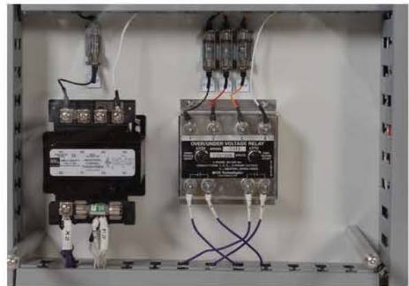
Close-Up of 3 Phase 400Hz AC Input Voltage Monitor to immediately disconnect Input Power to the UUTs if the Input Voltage is out of limits
